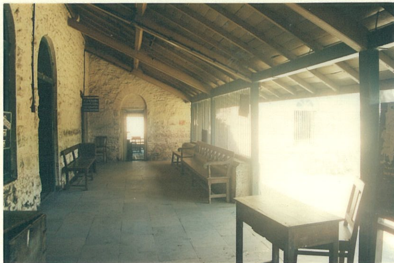
A wide verandah in timber frame fronts the main building in ashlar construction
