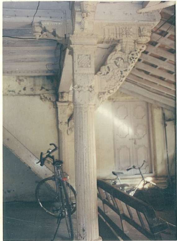
Carved timber columns with carved brackets in the front verandah of the ground storeyed wing
