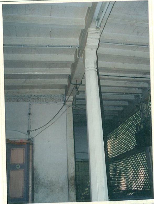
Carved timber column with carved brackets, in the front verandah
