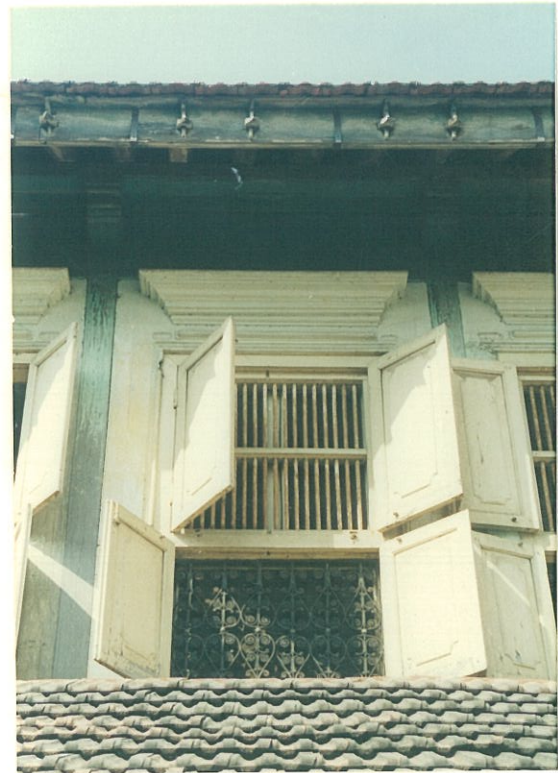
Full height window with elaborate cornice and architrave, over looking the front courtyard
