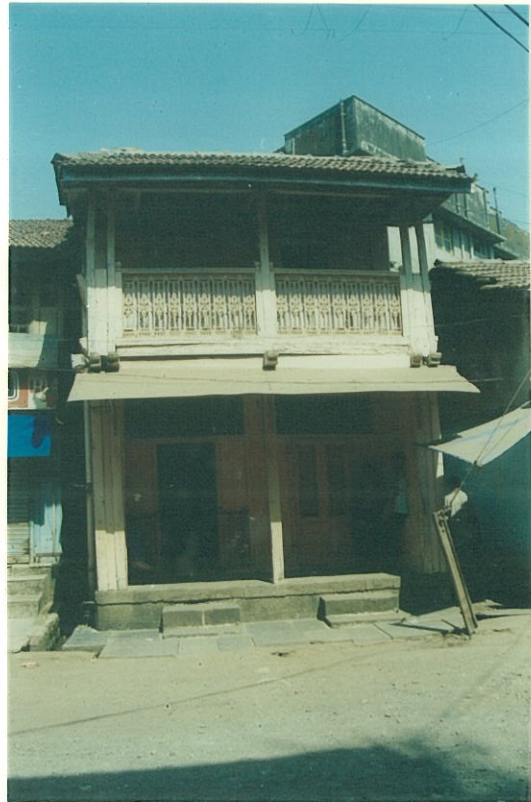
Front view showing the front verandahs with timber frame structure
