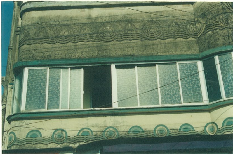
Art Deco mannerism seen on the façade like curved edges to the balcony and surface patterns
