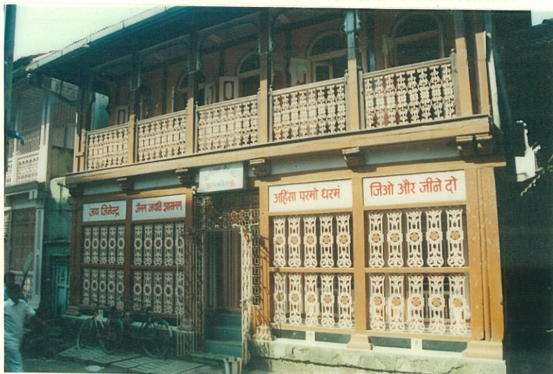
Detail of the front façade
