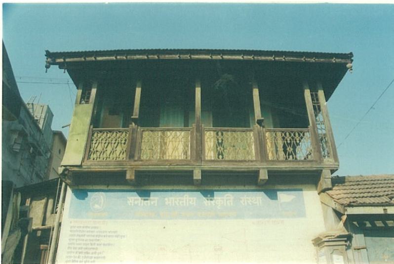
Balcony on timber brackets projecting from the blank ashlar wall of the kothar below
