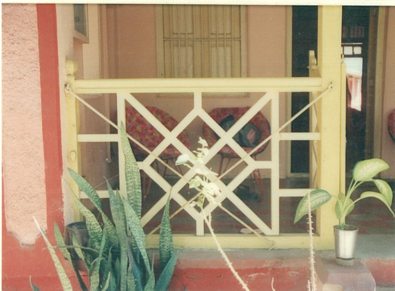
Detail of timber railing in the verandah
