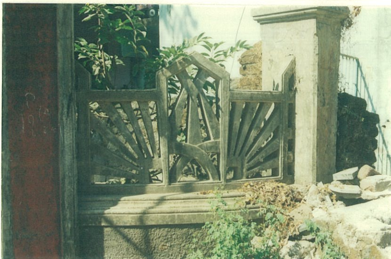
Detail of compound wall
