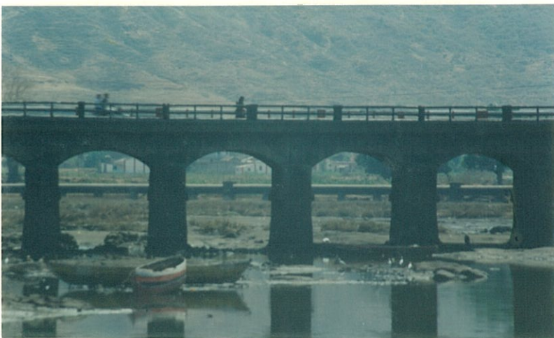
Close-up of the arches and piers
