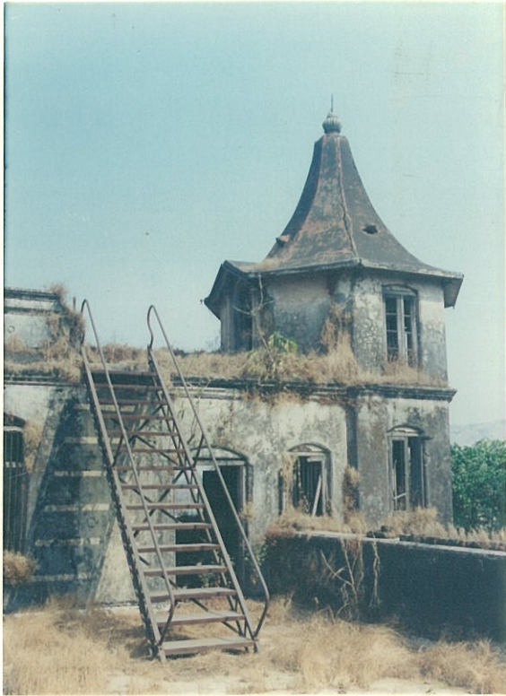
Octagonal corner tower with a pyramidal concrete roof
