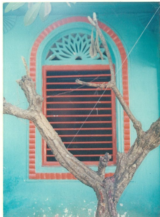
Detail of a window in front
