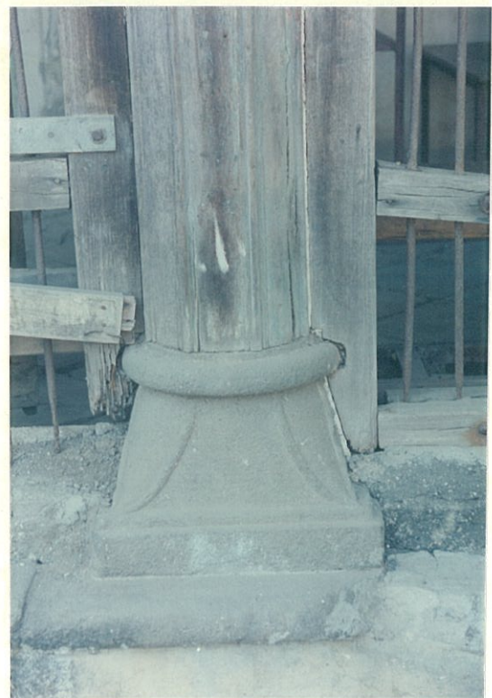
Carved timber column resting on a carved stone base
