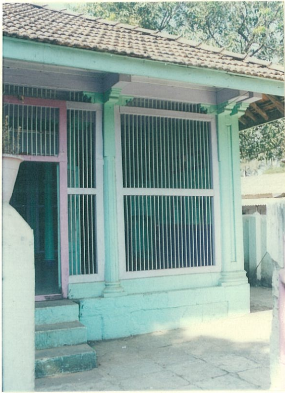
Typically Konkani style open front of the temple with TW framework and infill of vertical MS rod grill
