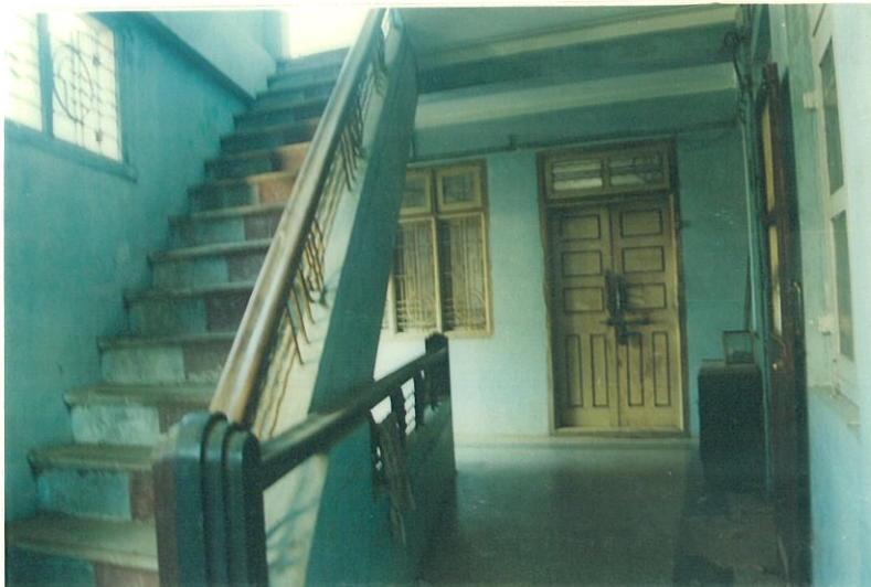
The skewed stairway creates an interesting corridor space
