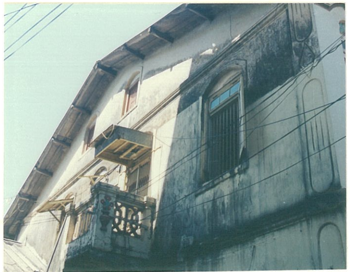
Side façade detail
