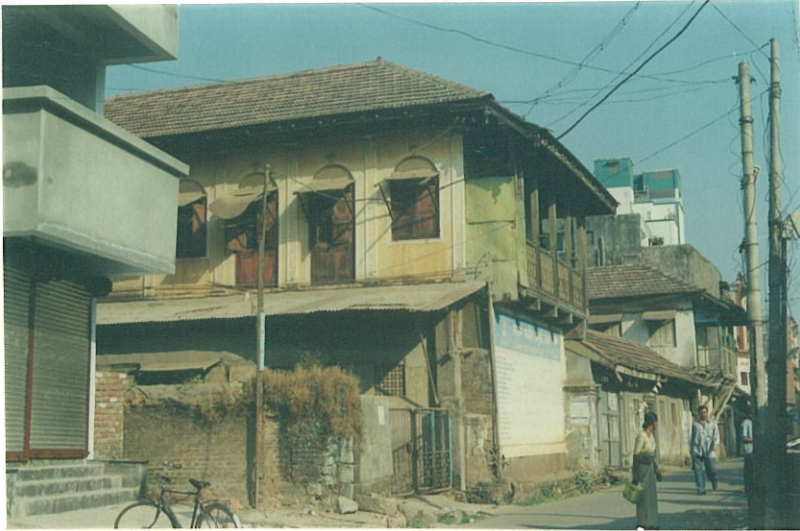
South corner view showing balcony projecting on the street
