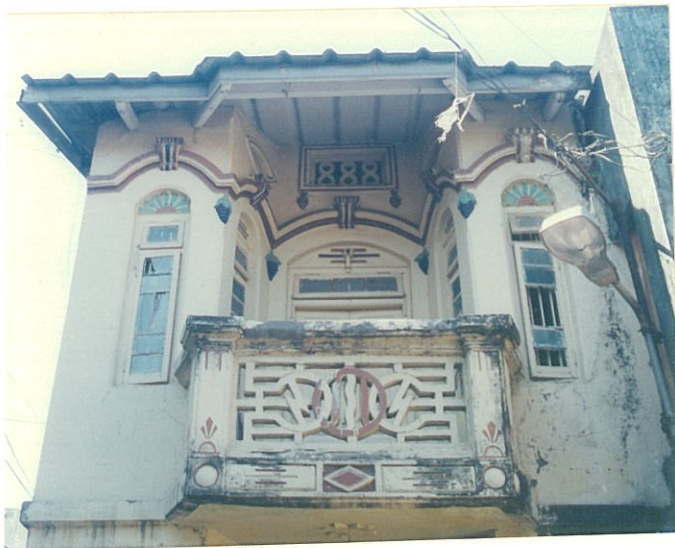
Front façade detail
