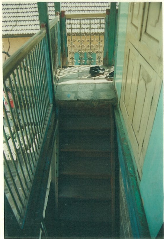
Straight flight timber staircase leads to balcony above
