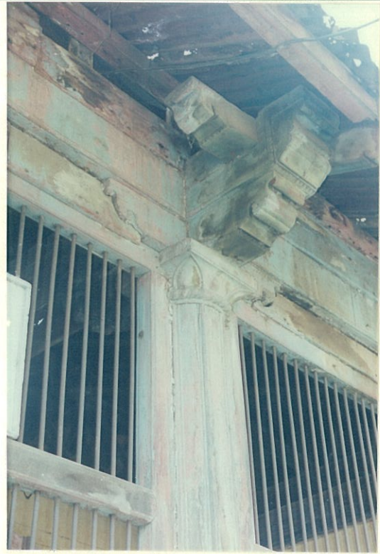
Timber column with carved capital and ornamental brackets
