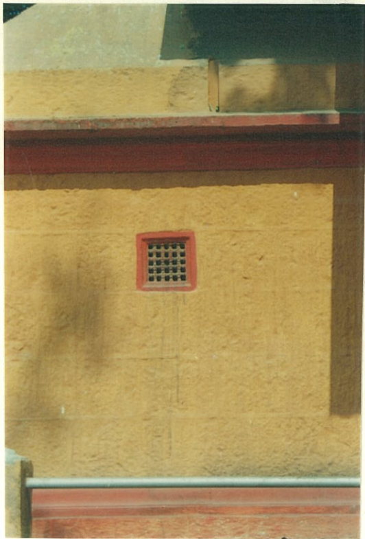
A small stone jaali in the ashlar wall of the garbhagriha
