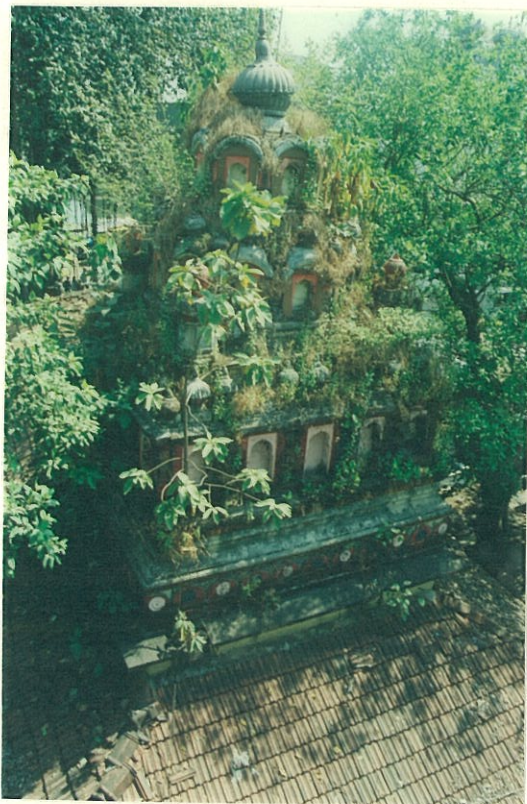
Peshwahi style shikhara over the central garbhagriha and TW lean-tos over the surrounding pradakshina
