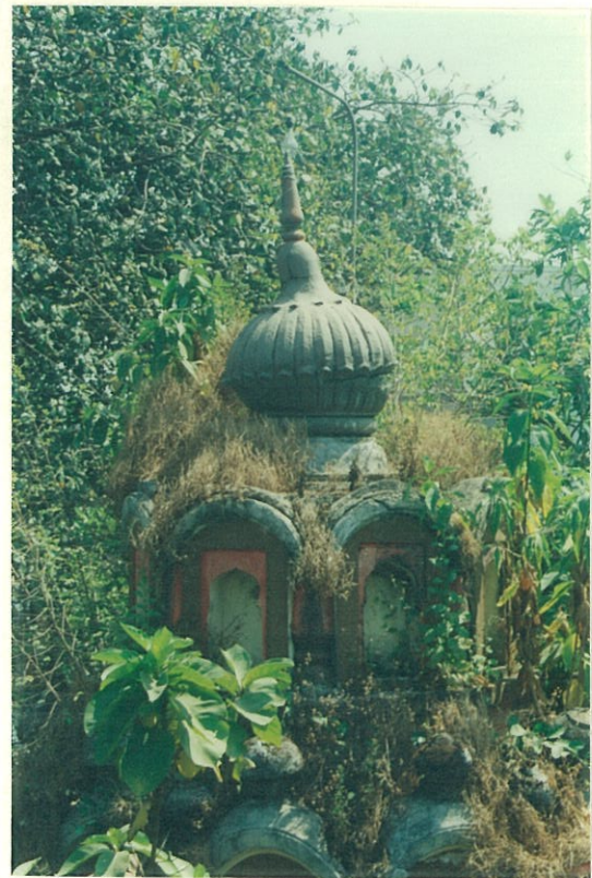
Tiered arched niches in brick and stucco with a carved amalaka at the pinnacle
