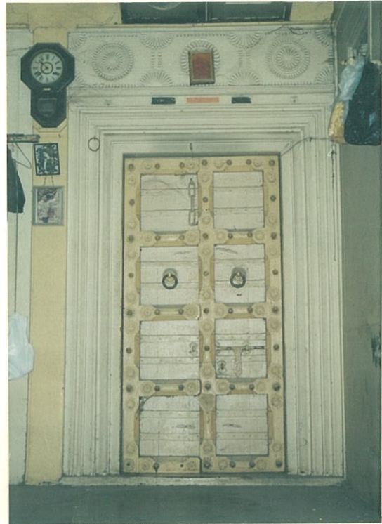
One of the many heavy timber doors with elaborate architrave and brass knobs and knockers
