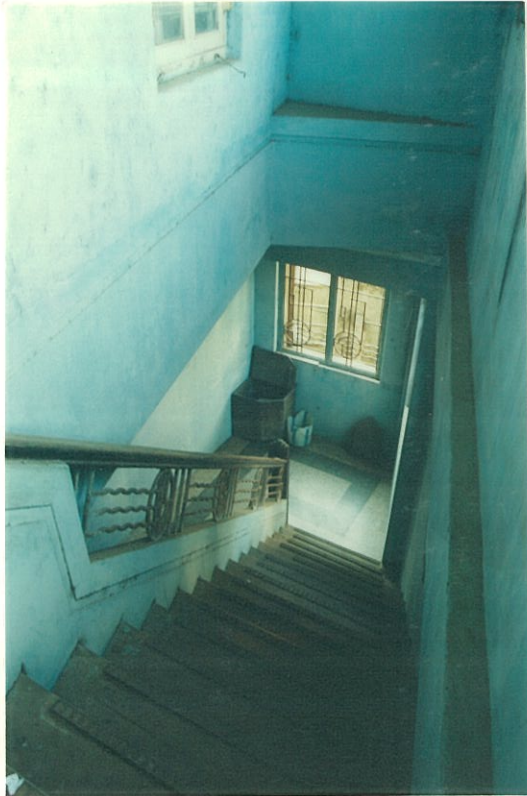
The stairway is skewed with respect to the building grid. Art Deco design seen in the railing
