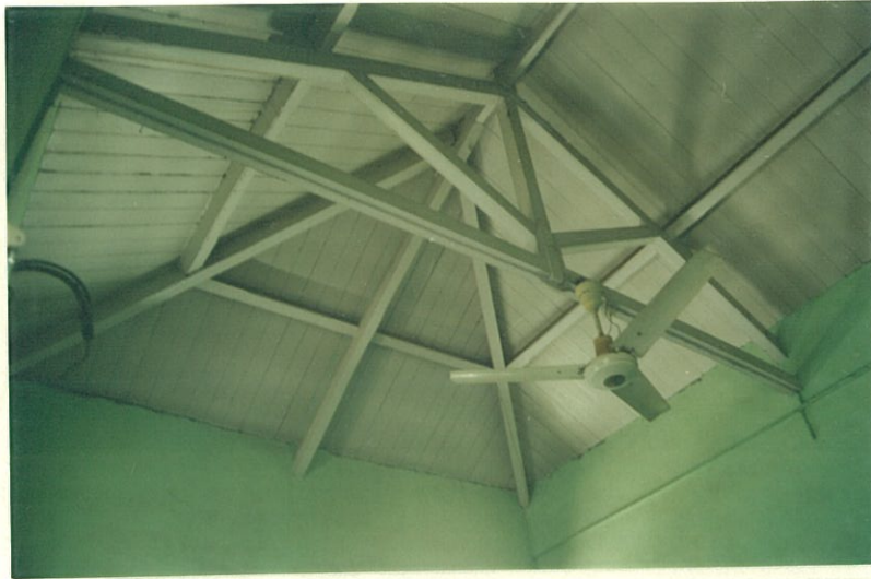
View of the King-post roof truss
