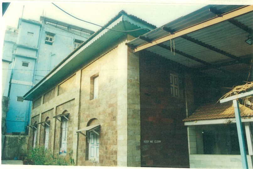
Courtyard side view of the building with the original porch seen below the temporary roof cover
