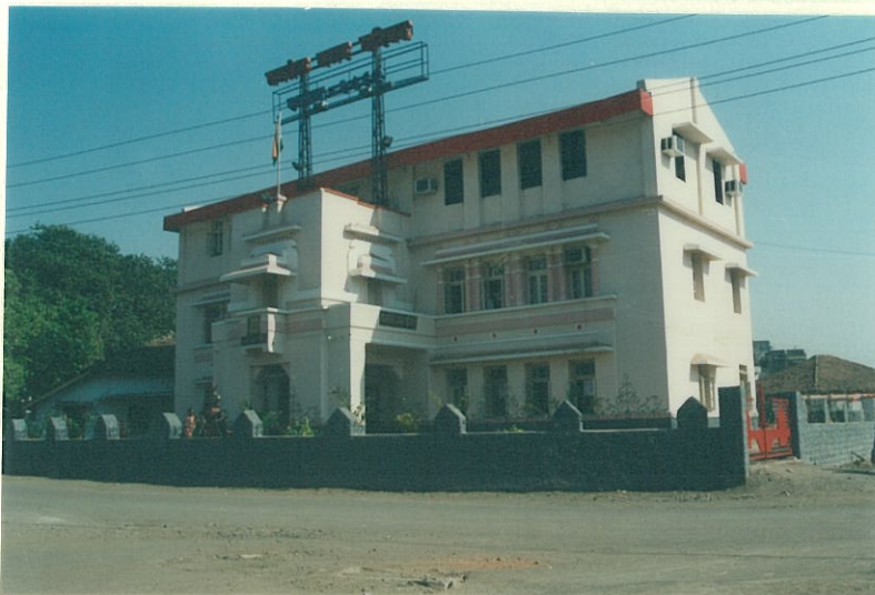
Front view of the building
