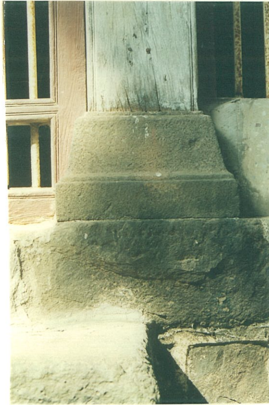
Timber post resting on a moulded stone base
