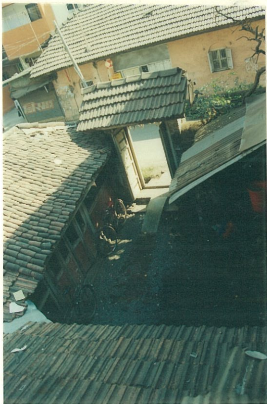
Top view of the courtyard and Dindi Darwaza
