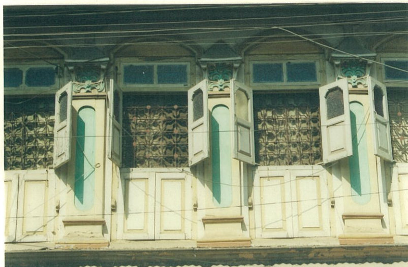
Detail showing Baroque articulations of the plastered bays
