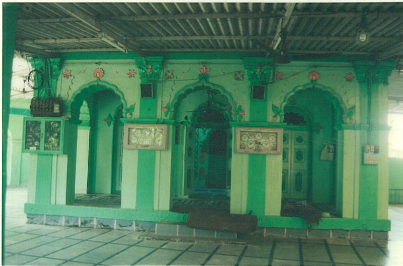
Arcaded verandah fronting the prayer hall showing articulation in stucco
