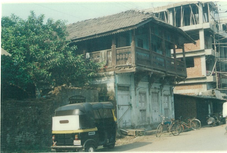
The corner view showing upper floor corridor turning the corner and becoming a projecting balcony on the street.
