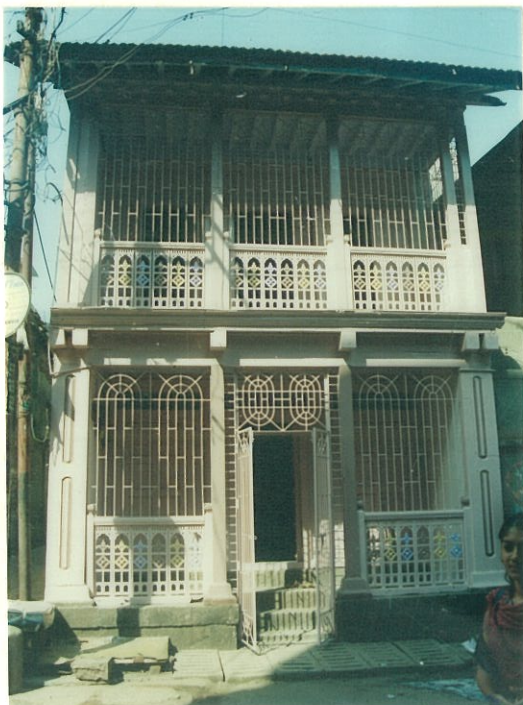
View of the front façade and detail of verandah
