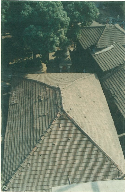
Top view of the premises from behind. The courtyard in front of the temple can be seen in the background
